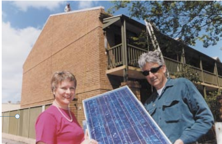
City resident, Christina Crosby, installs solar panels to reduce energy consumption.
