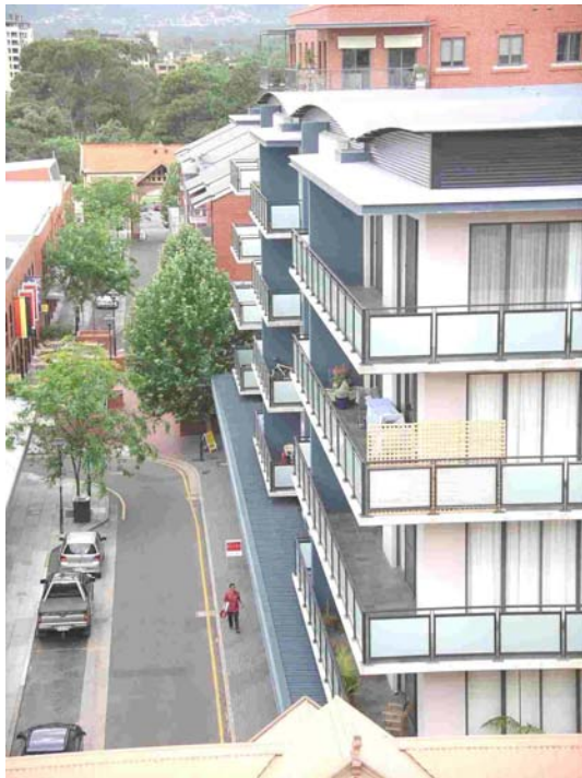
The Garden East development on the site of the former Adelaide Fruit and Produce Exchange has demonstrated the attractions of apartment living in the East End.
